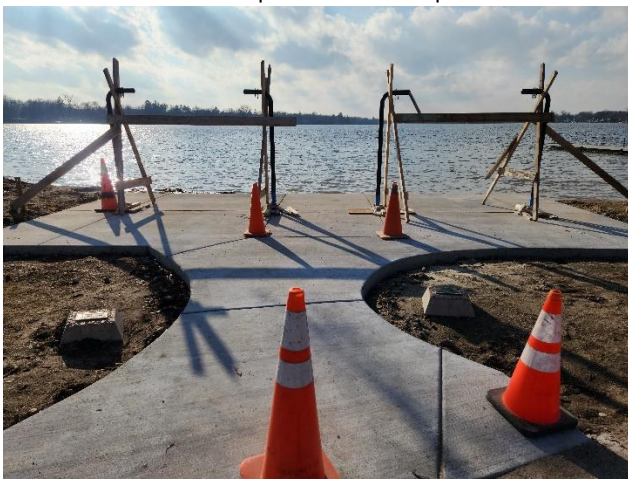
Swing Bench Posts Installation
