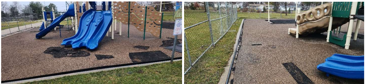
Repairing the existing rubber surfacing and attaching the nailer boards.
