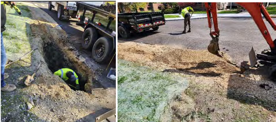
Excavating to find the line Backfilling the hole
