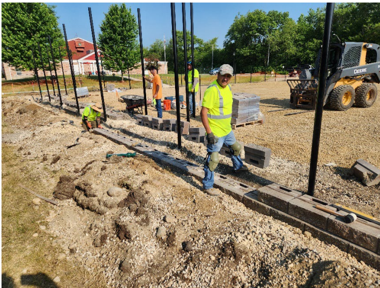
Retaining Wall Installation and Geo-Grid tie-in.
