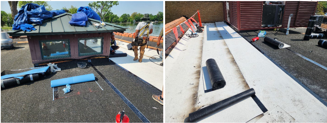
Work in process
