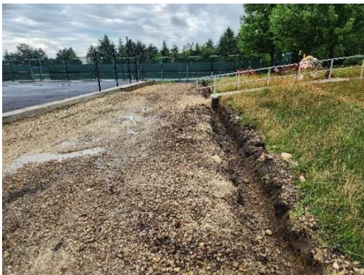
Trench for concrete curb.
