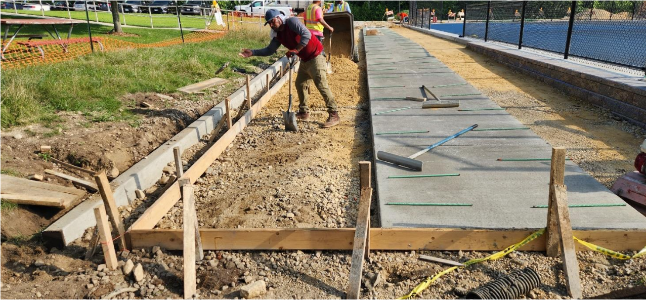
Concrete installation work
