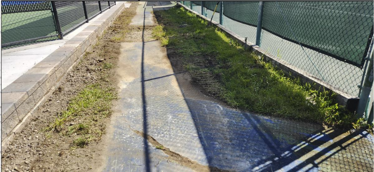
View of Asphalt Pathway Looking East
