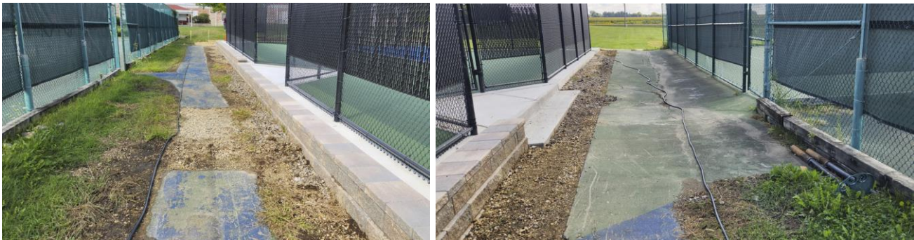
Photos of Existing Conditions, views looking west / east.
