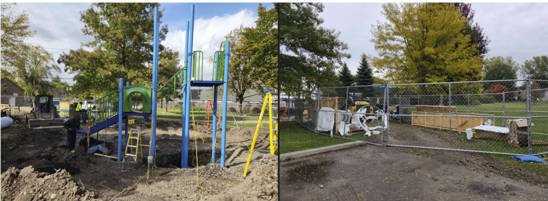
Kamijima Playground – Installation in process.
