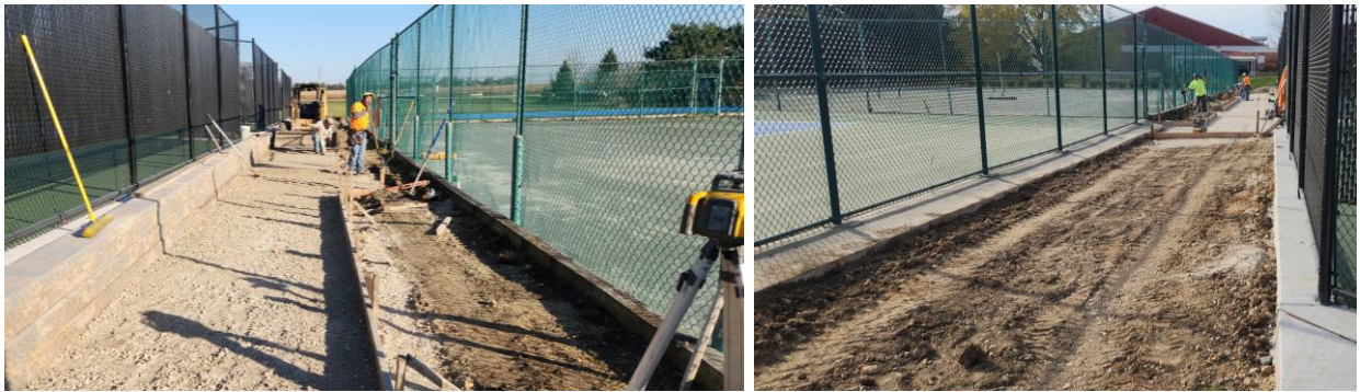
Construction In Progress
