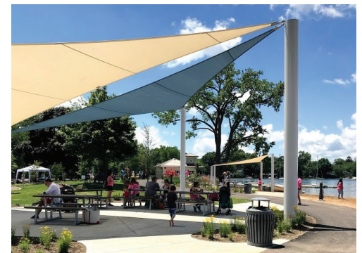
Main Beach Shelter #6
