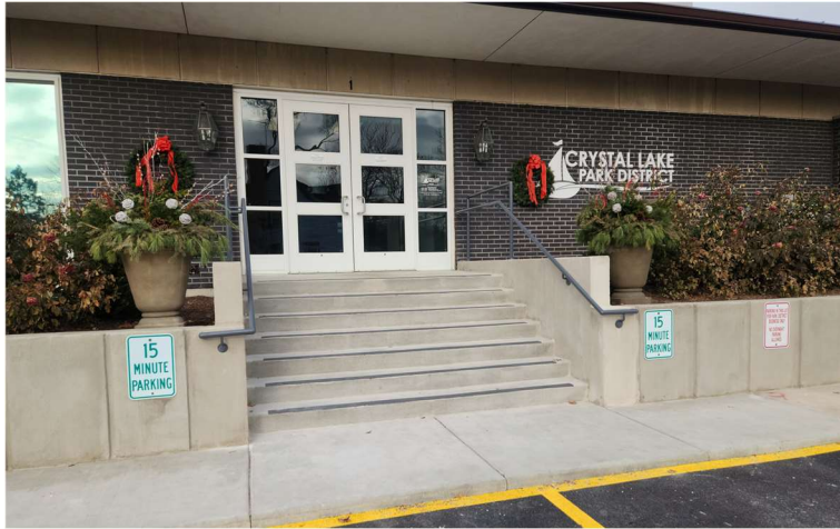
Installed Handrails
