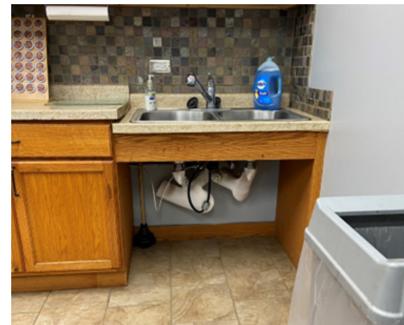
Accessibility improvements at break room sink
