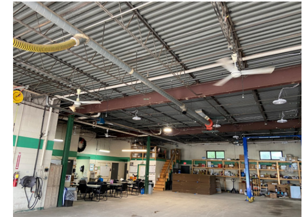
Building structure as viewed from newer portion of interior
